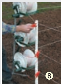
Attach the cross-connections approx. every 200 m
