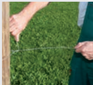
2. Wind the free end of the wire around the tension wire 3 times
