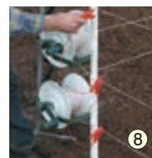
8 Attach the cross-connections approx. every 200 m
