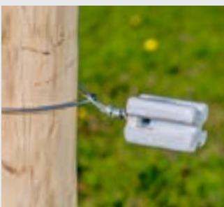
5. The completed knot – the tension runs centrally through the insulator
