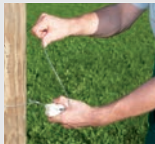
3. Feed the free end of the wire into the strain insulator
