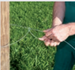
1. Place the wire around the post and form a loop
