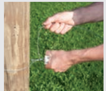
4. Wind the free end 5 times around the tension wire
