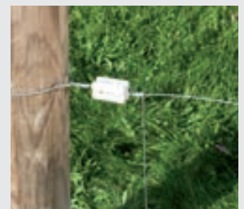
8. Leave the free end long to allow for cross-connection
