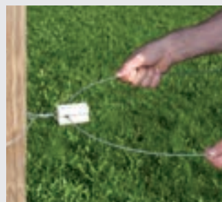
6. Pull the fence wire through the insulator
